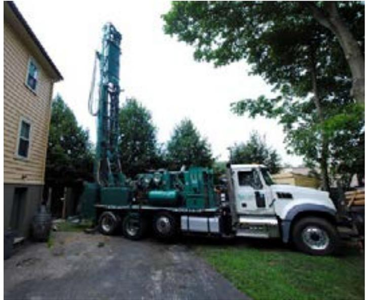
After conducting an energy audit that showed the house was poorly insulated and inefficient, Achieve increased insulation in the attics, walls, and basements prior to installation. The energy efficiency upgrades allowed Achieve to install a smaller system, lowering the project costs and operating expenses for the homeowners. The ground-source heat pump system consists of two heat pumps and two bore holes, each with a depth of 380 feet.
